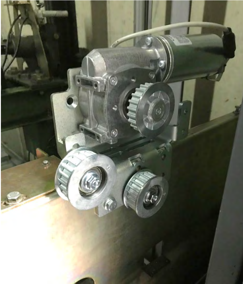
ill.2: TSG motor mounted at IGV door
