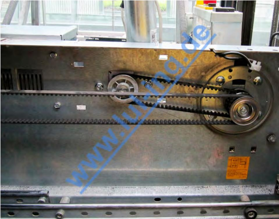
**Fig. 9: fully mounted TSG drive with replaced toothed belt**
