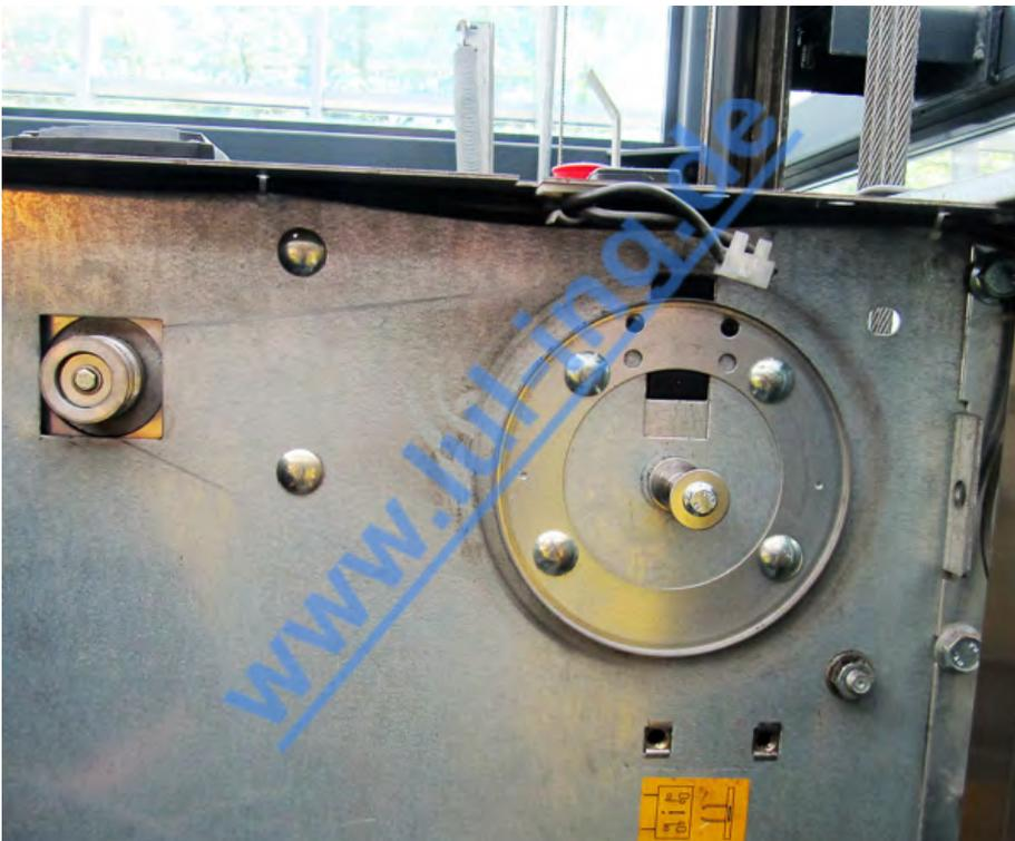
**Fig. 4: dismantled tooth belt pulley, mounted new axis**
