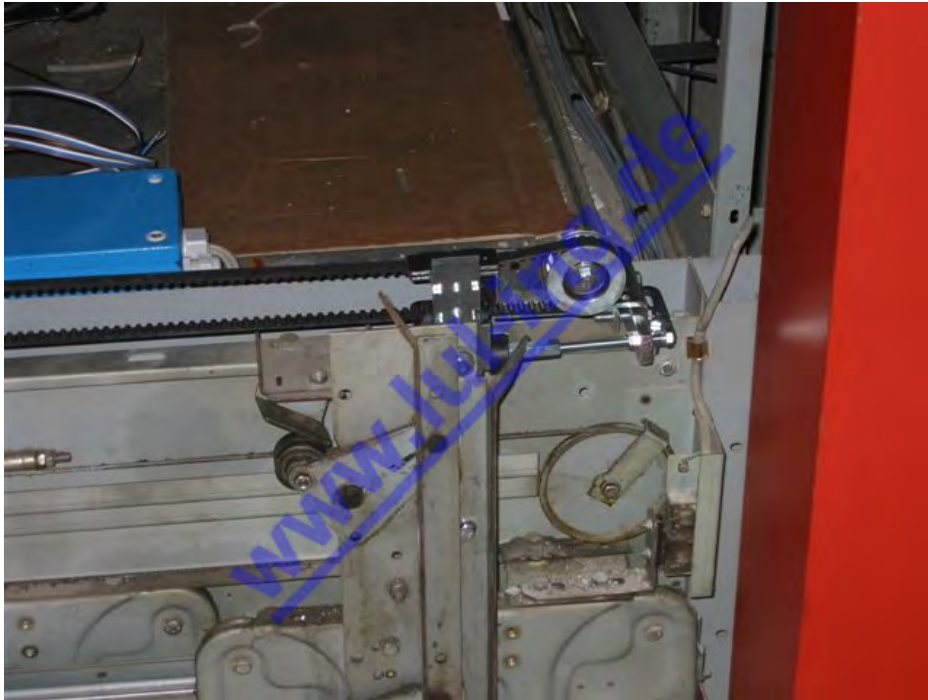
Fig. 5: KONE ADM - counter roller
