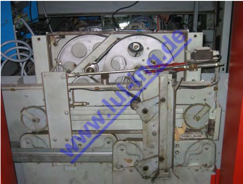
Fig. 1: KONE ADM before conversion
