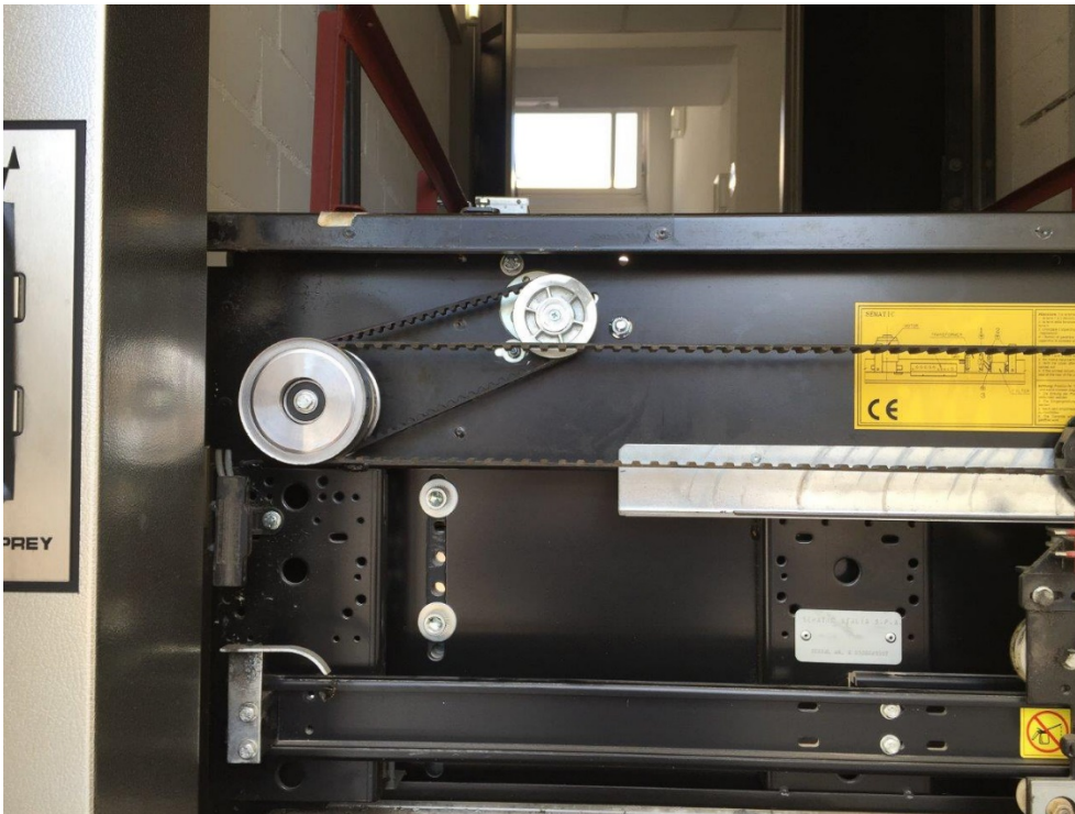
Fig. 16: fully assembled door operator with TSG (telescoping right opening)
