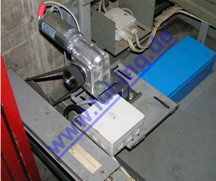
Fig. 6: Thyssen M2 after conversion: TSG drive
