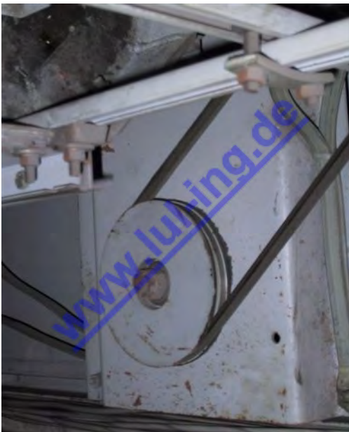
Fig. 5: Thyssen M2 before conversion: version with V-belt pulley
