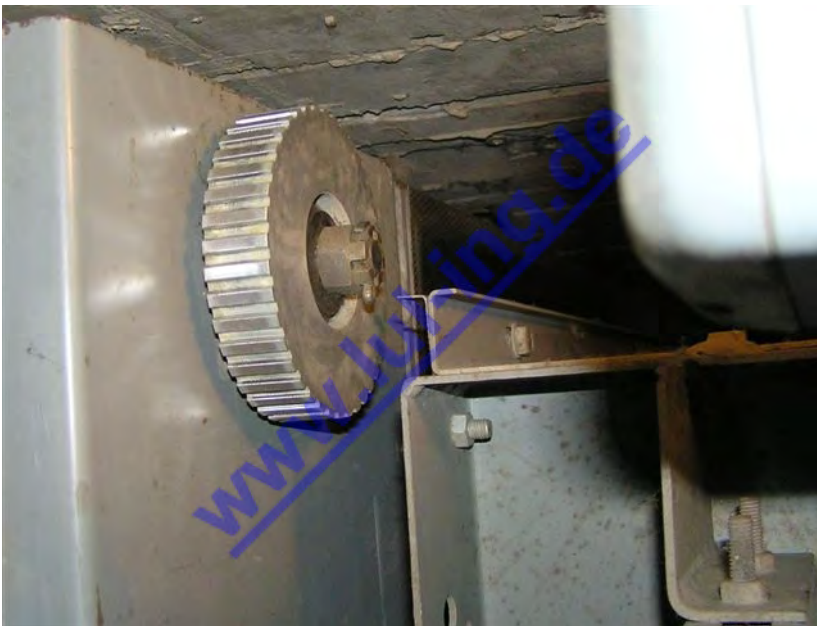
Fig. 3: Thyssen M2 before conversion: Version with old toothed pulley
