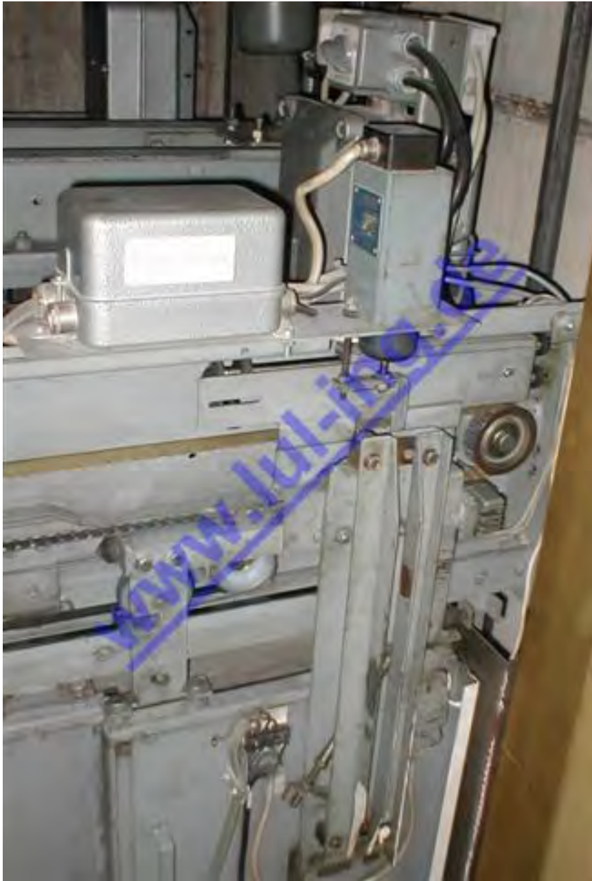
Fig. 1: Thyssen M2: Closing side with magnet for skate
