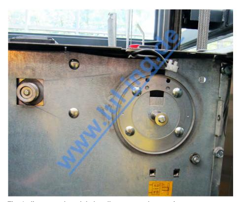
Fig. 4: dismounted tooth belt pulley, mounted new axis
