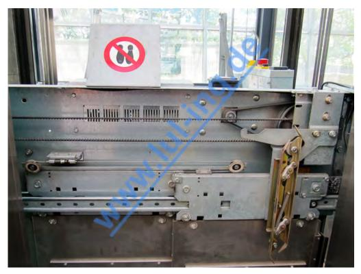
Fig. 1: Schindler Varidor 50 original (here: telescoping left)
