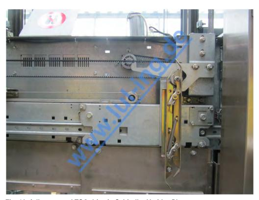
Fig. 10: fully mounted TSG drive in Schindler Varidor 50
