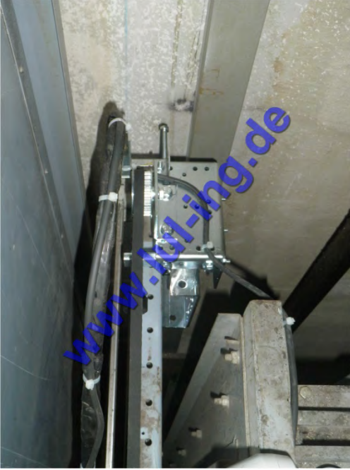
Fig. 5: TSG deflection roller
