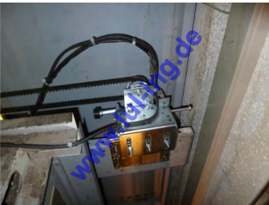
Fig. 6: TSG deflection roller
