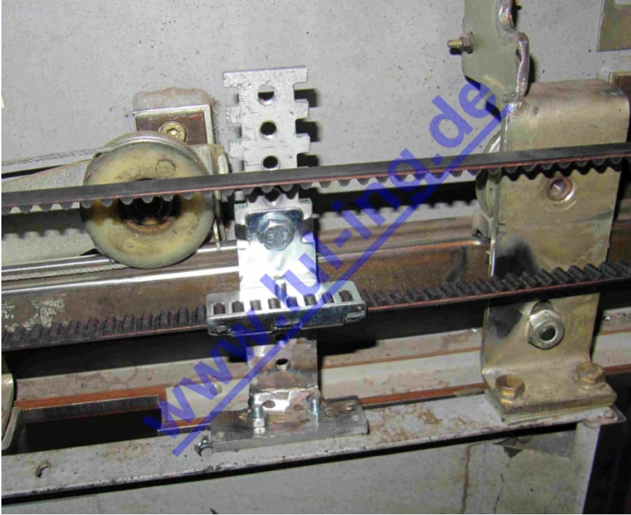
Fig. 13: TSG in Rathgeber – door panel carrier on door panel
