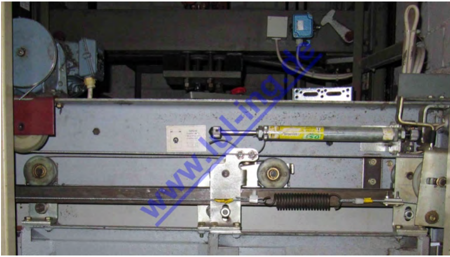
Fig. 1: Rathgeber door machine with wire cable (original)
