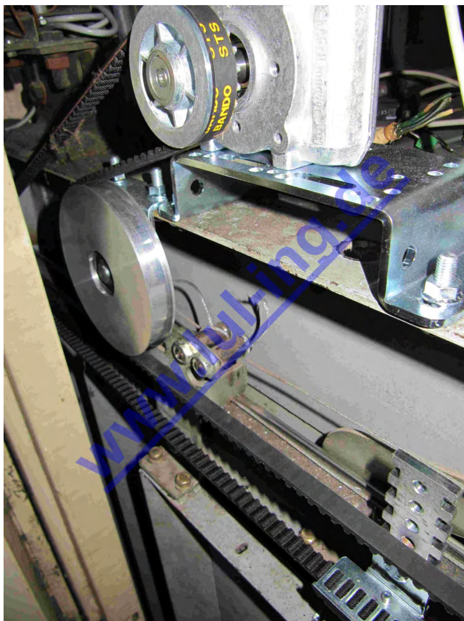
Fig. 5: TSG drive with deflection roller - installed in door machine
