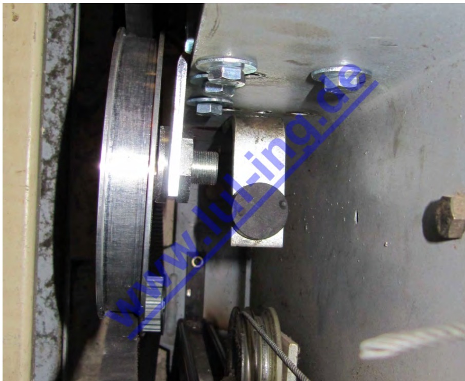
Fig. 6: TSG stop - installed in door machine
