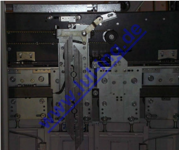
Fig. 1: Monitor for 99VF door machine, original (here: centrally telescoping)
