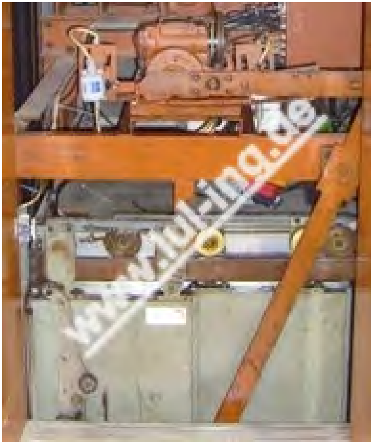
Fig. 1: Haushahn door drive TS54 before conversion
