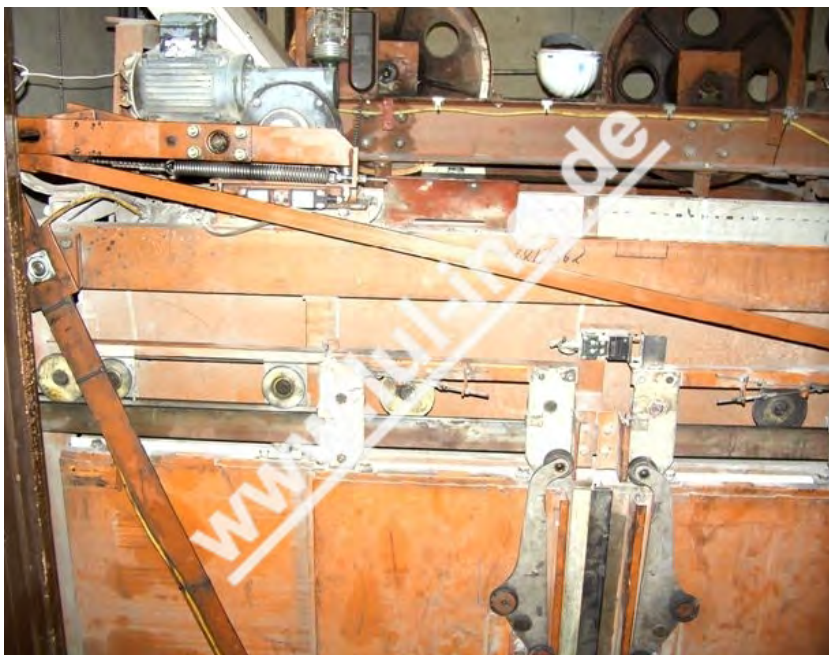
Fig. 2: Haushahn door drive TS54 before conversion
