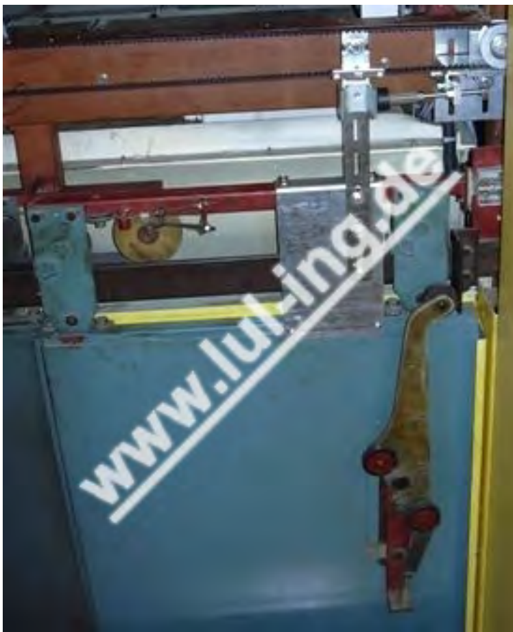
Fig. 4: Haushahn door drive TS54 after conversion with TSG
