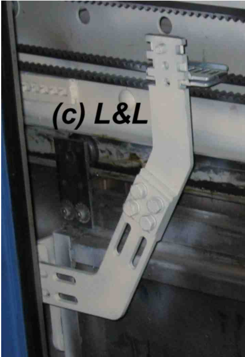
Abbildung 17: coupler on the slow door panel (here: telescoping left)
