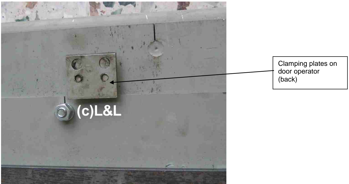
Abbildung 7: clamping plates on new door operator
