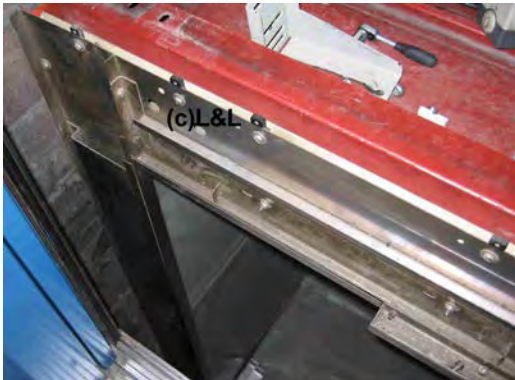
Abbildung 3: car P8K without door operator – right side (TL)
