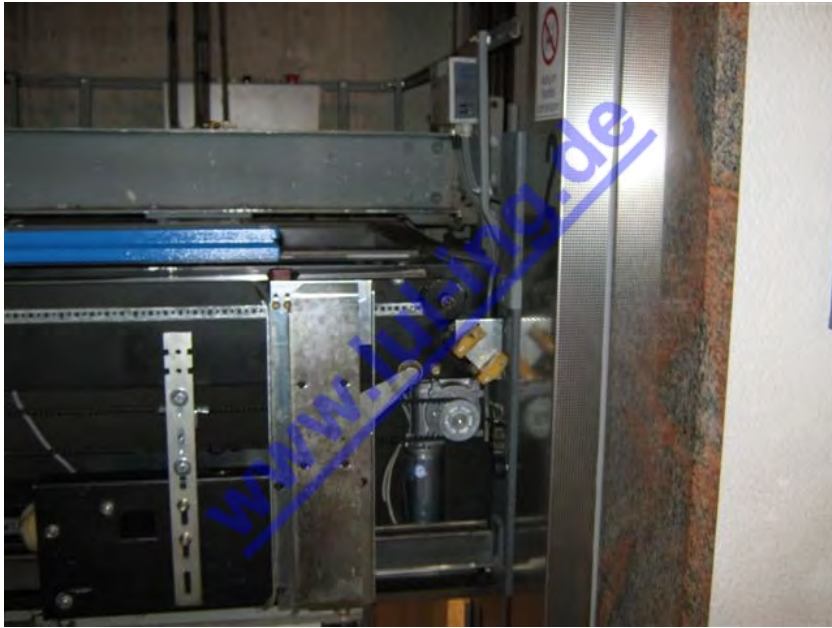
Fig. 3: Door machine with TSG after conversion is complete - closing side
