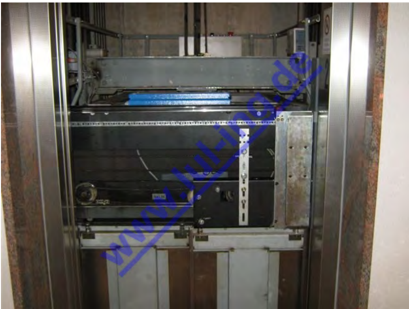
Fig. 2: Door machine with TSG after conversion is complete
