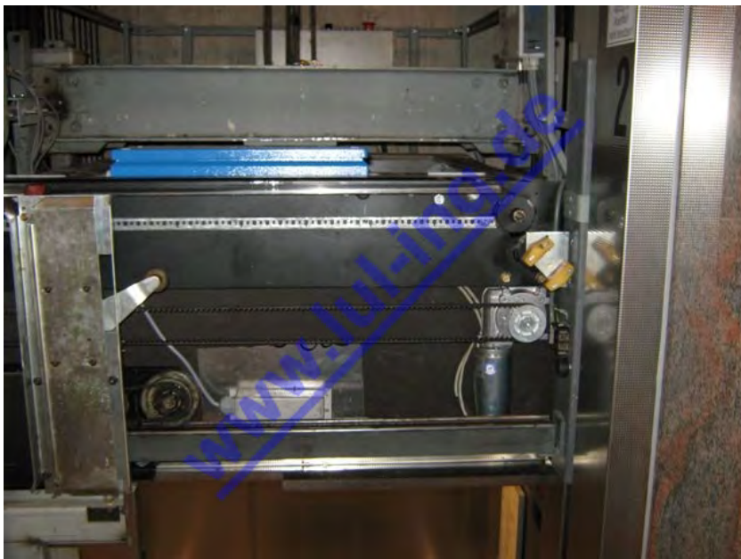
Fig. 4: Door machine with TSG after conversion is complete - closing side
