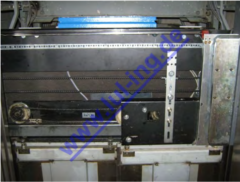
Fig. 5: Door machine with TSG after conversion is complete
