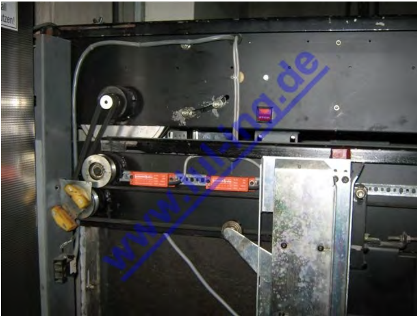
Fig. 1: Schmitt & Sohn door drive before conversion
