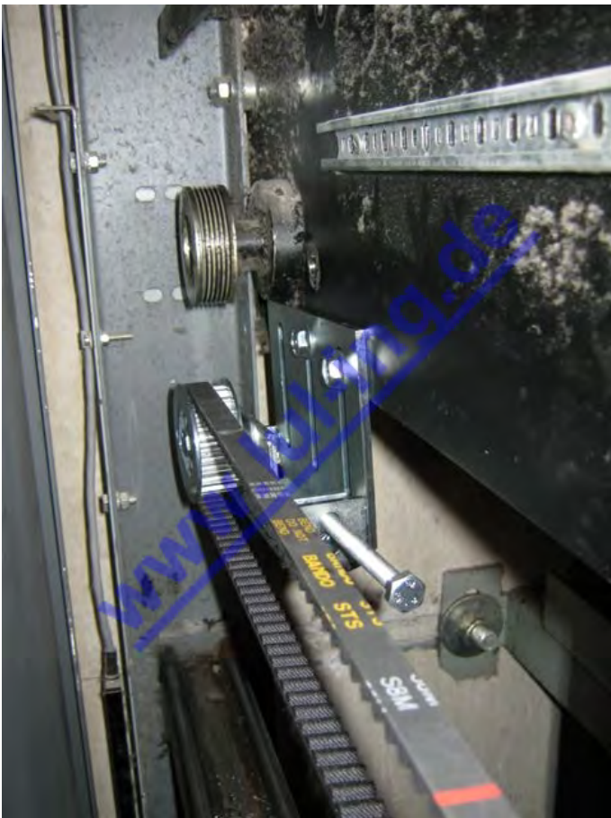
Fig. 6: Door machine with TSG after conversion is complete - opening side
