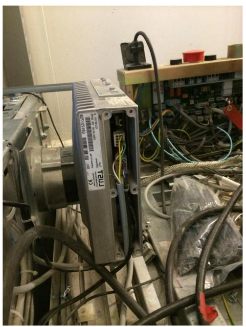
Abb. 5 LUST door operator with LON bus
