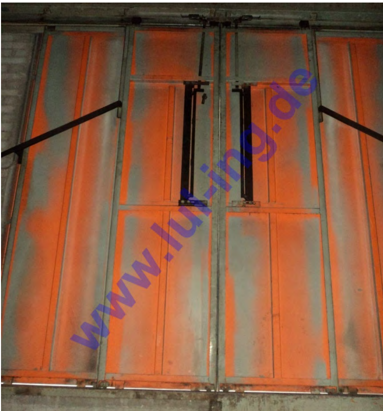
Abb. 4: original Schindler QKS6 / QKS7 Schachttür ZT
