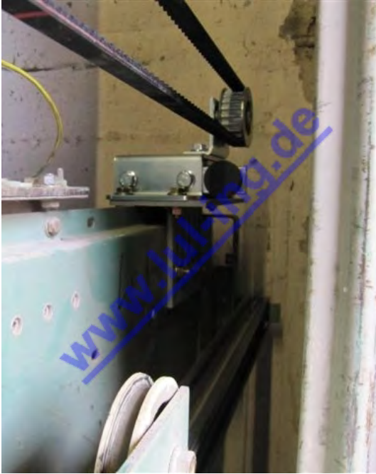
Fig. 5: TSG deflection roller
