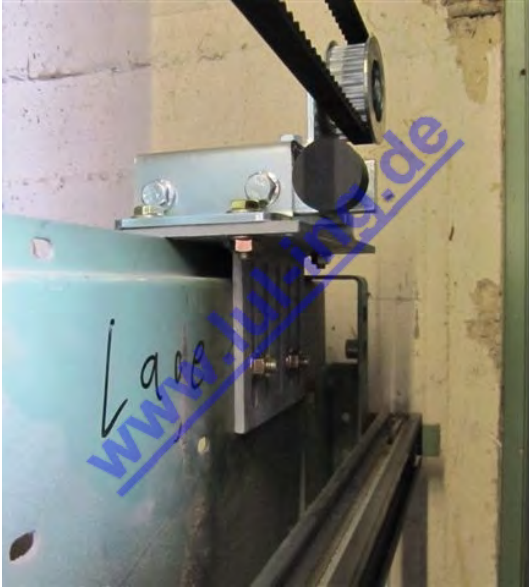
Fig. 7: TSG deflection roller
