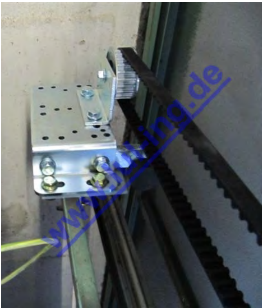
Fig. 6: TSG deflection roller
